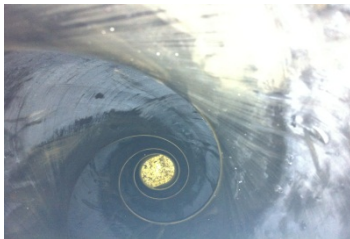
Figure 21: A stator in good internal condition
